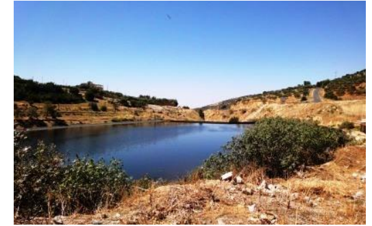
Salt, Jordan – Waste Water Treatment Plant, basin
