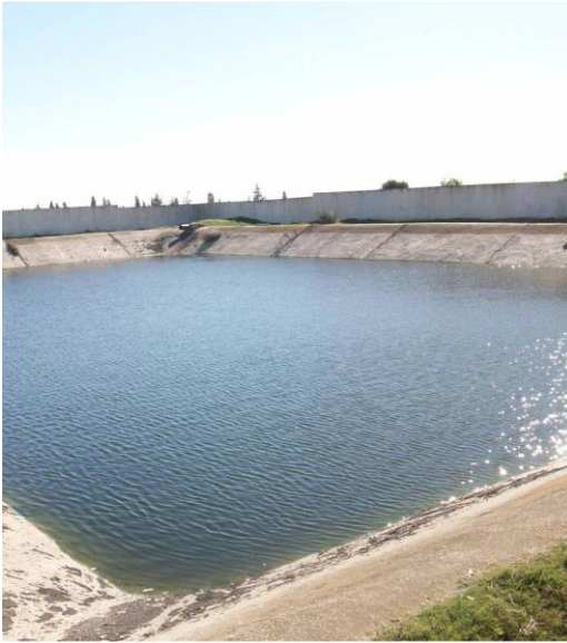
Nabeul, Tunisia – Waste Water Treatment Plant, basin
